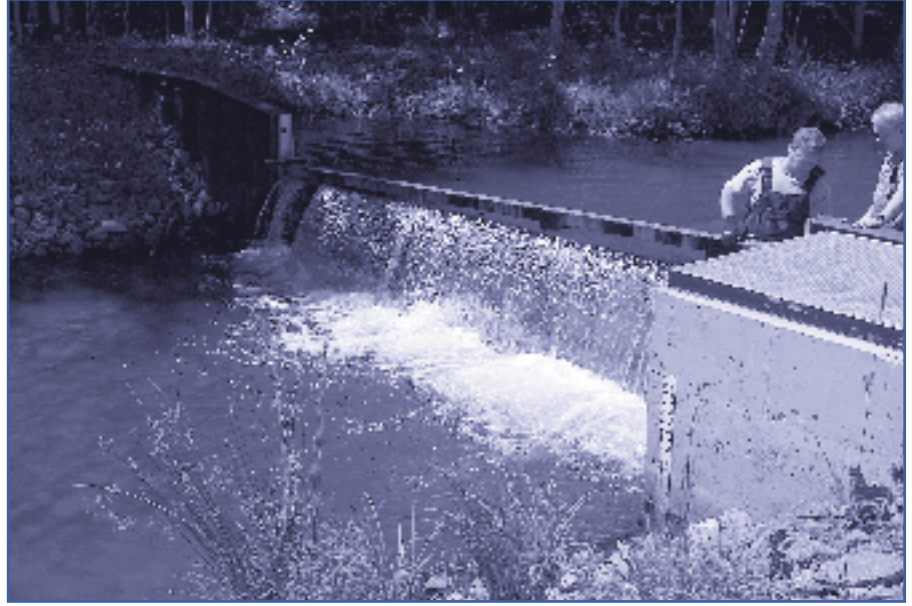
Sea lamprey barriers, like this one on Michigan's Little Carp River, prevent lamprey from reaching spawning grounds to reproduce.
