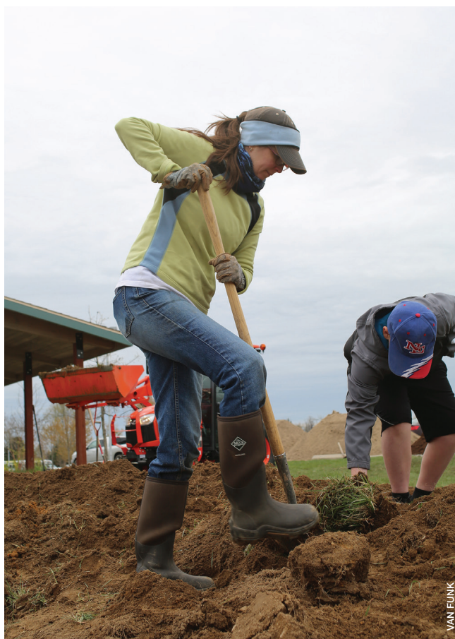
Extension faculty assists in stormwater management construction.
