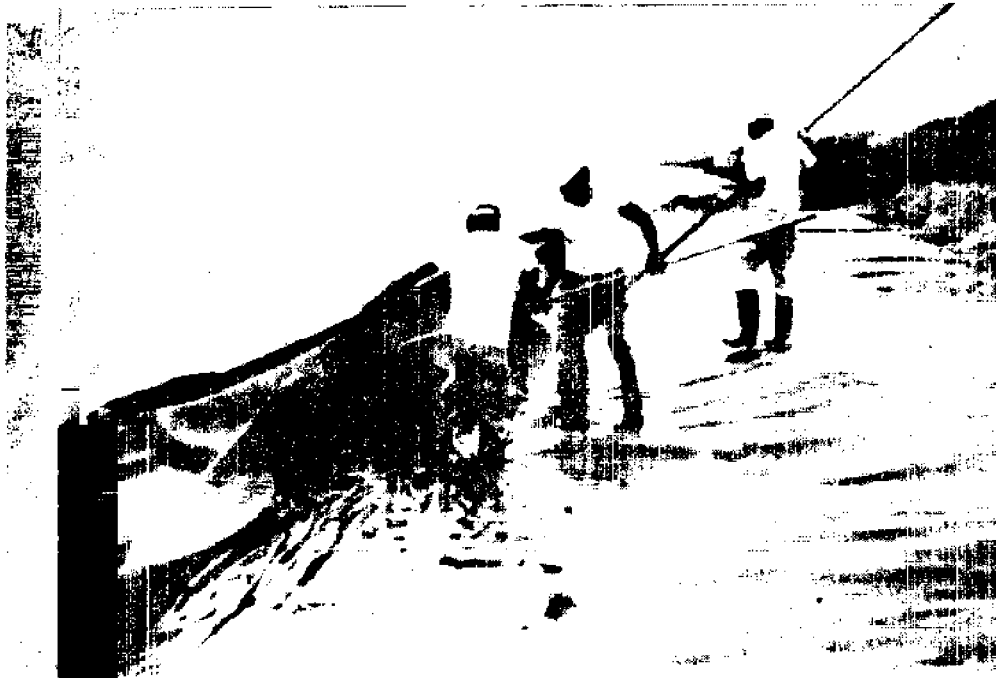
Figure 5. Launching and spreading fabric on advancing mud wave (from east to west)
