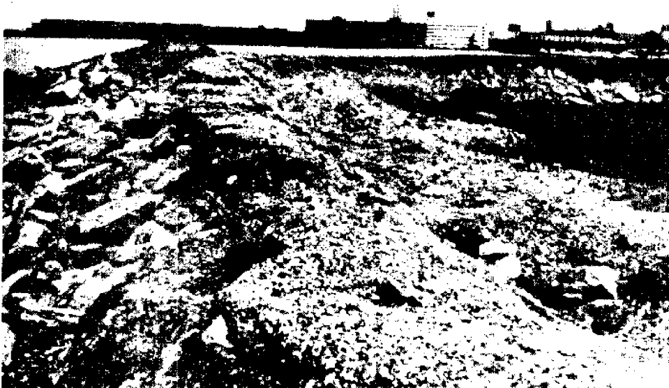
FIG. 20.--Displacement and Loss of Stone Protection on Dike Due to Overtopping
