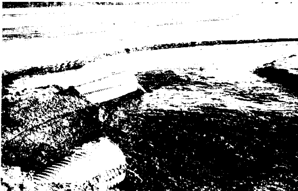
FIG. 18.--Erosion From Outfall Discharge (Note Loss of One Section of Pipe)
