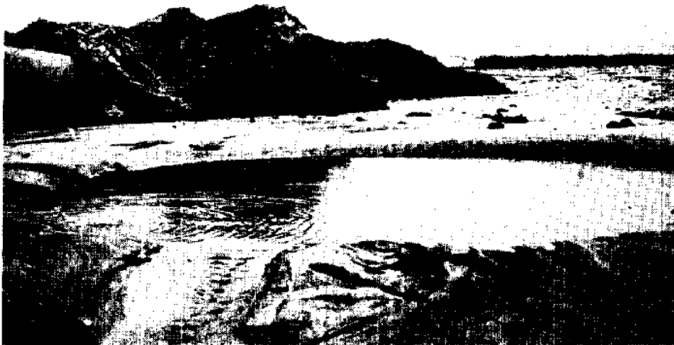
FIG. 17.--Depression at Discharge Point Formed By Impact of Pumped Material
