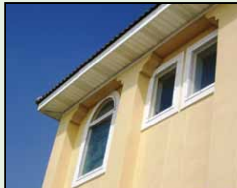
Figure 23. Flat impact polycarbonate panels are installed directly over windows of a coastal home. This window covering provides excellent storm protection with minimal aesthetic impact. Source: Roll-a-way/QMI.
