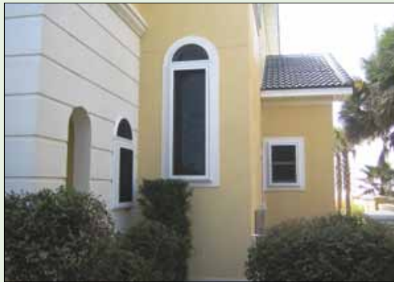
Figure 22. In-place stainless steel impact screen protecting several windows of a coastal residence. This system requires no deployment and provides shade.
