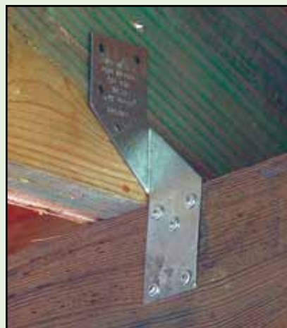
Figure 13. A hurricane clip installed during new construction. A hurricane clip is required for each truss-rafter that is hidden from view upon completion of the structure.
