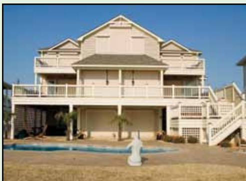
Figure 16. Coastal home protected with roll-down shutters on all windows and doors. The shutter is held in place by vertical guide tracks and can be deployed manually or with an integrated electric motor. Source: Roll-a-way/QMI.
