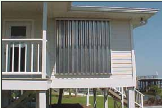
Figure 21. These 0.050 gauge aluminum storm panels offer cost-effective storm protection. In this example, panels slip into a track above the window and secure onto a bottom track using wing nuts. Source: Roll-away/QMI.
