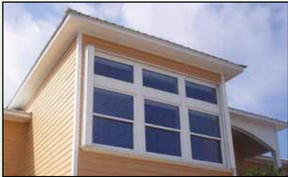
Figure 17. Accordion shutter (shown in open position) installed over a large window group of a coastal home. Shutter has been installed to allow deployment from inside the home. Source: Roll-a-way/QMI.
