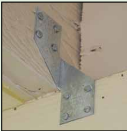
Figure 33. This is an example of retrofitting an existing house, originally built without hurricane clips. The popular H3 clip is used here; four nails attach the clip to the roof (truss-rafter) and four more nails attach to the wall or top plate below. For a retrofit, the clips are exposed on the outside of the house; therefore, both the clip and fasteners should be corrosion-resistant and painted to blend with the exterior of the house. With the correct clip and nails, you could perform the work or, if you prefer, hire a licensed contractor.
