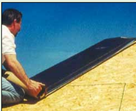
Figure 14. Synthetic underlayment is typically made from polypropylene, polyester, or fiberglass fabric that weighs less than felt building paper, and withstands exposure to varying weather conditions. Source: Carlisle Coatings & Waterproofing.
