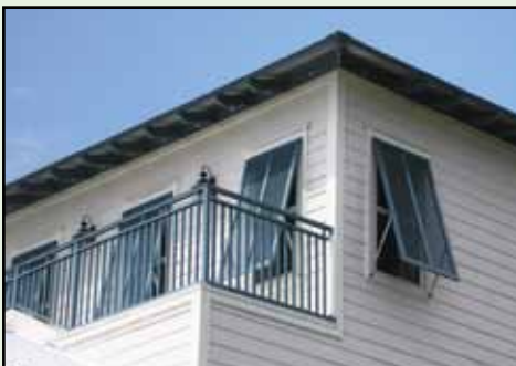
Figure 18. Bahama shutters made from durable extruded aluminum components add "Island" flair to a home and provide effective opening protection. Source: Roll-a-way/QMI.
