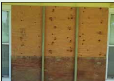
Figure 28. For larger windows, such as this sliding glass door, two 2 by 4s face outside and are oriented with the narrow end against the plywood. The fastening screws attach from the plywood into the 2 by 4.
