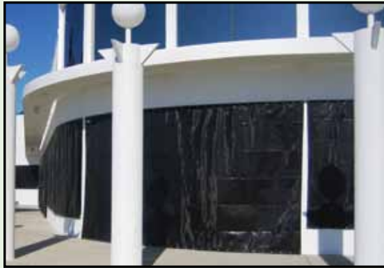
Figure 24. Polyethylene basket-weave fabric windscreen deploys directly over the ground floor windows of a coastal home. Source: Roll-a-way/QMI.
