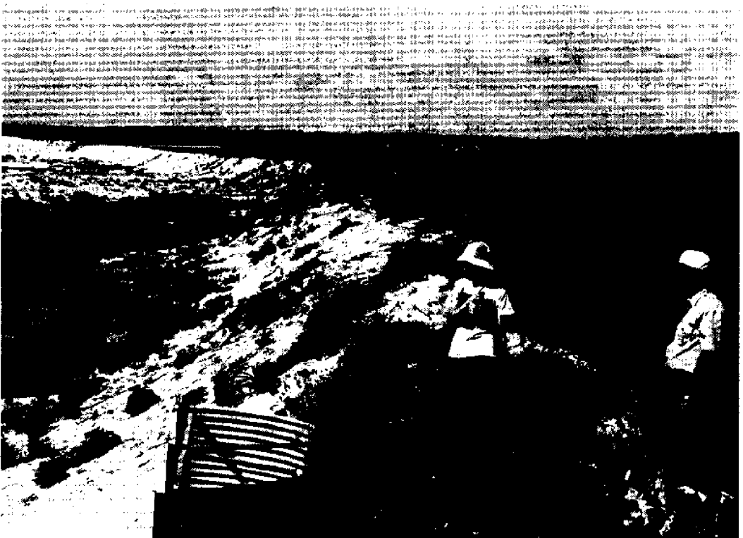
Fig. 11. One-year old dike showing invasion of plants.
