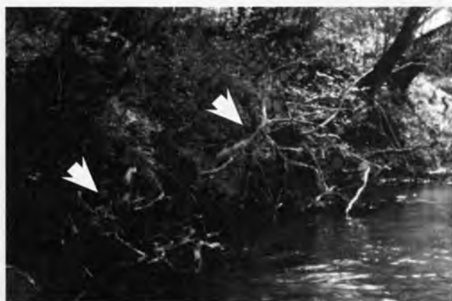
Figure 2. Root wads after installation.
