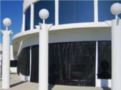
Figure 4-18. Polyethylene basketweave fabric windscreen deploys directly over ground floor windows of coastal home. Source: Roll-a-way/QMI
