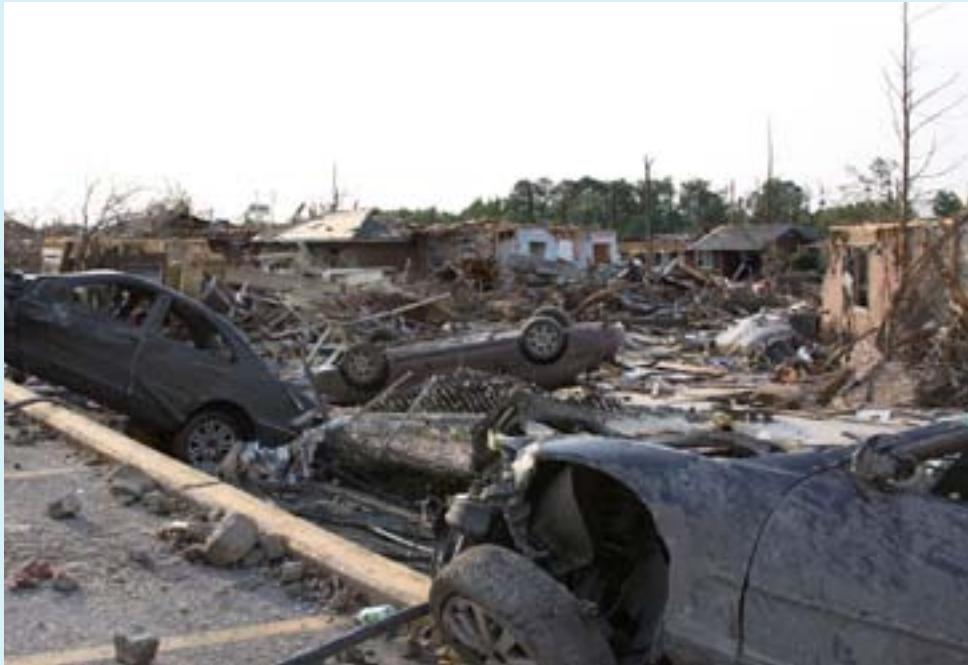
Figure 2-1. Major tornado damage in Tuscaloosa AL, in April 2011. Source: NOAA www.oceanservice.noaa.gov
