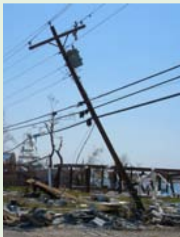
Figure 4-25. Downed or damaged power lines in a residential area can pose a serious danger to public safety. Source: U.S. EPA
