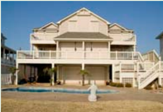
Figure 4-10. Coastal home protected with roll-down shutters on all windows and doors. The shutter is held in place by vertical guide tracks and can be deployed manually or with integrated electric motor. Source: Roll-a-way/QMI
