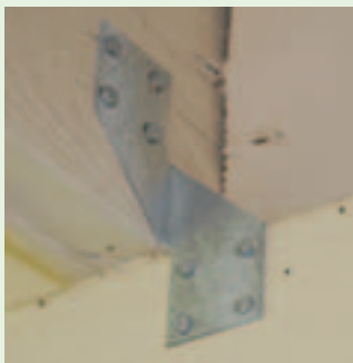
Figure 4-27. This is an example of retrofitting an existing house originally built without hurricane clips. The popular H3 clip is used here; four nails attach the clip to the roof (truss-rafter) and four more nails attach to the wall or top plate below. For a retrofit, the clips are exposed on the outside of the house; therefore, both the clip and fasteners should be corrosion resistant and painted to blend with the exterior of the house. With the correct clip and nails you could perform the work or, if you prefer, hire a licensed contractor.
