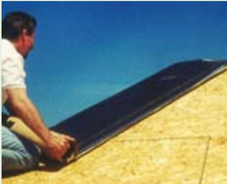
Figure 4-8. Synthetic underlayments are typically made from polypropylene, polyester or fiberglass fabric which weighs less than felt building paper, can be manufactured with anti-slip surfaces and can withstand exposure to the elements for six months. Source: Carlisle Coatings & Waterproofing
