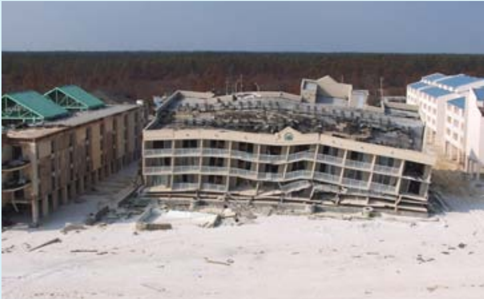
Figure 2-5. Storm surge associated with Hurricane Ivan caused damage to properties in Gulf Shores, Alabama. Source: AEMA
