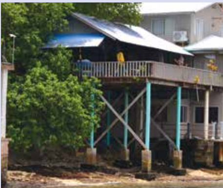
Figure 4-40. This house in Majuro was elevated to prevent damage from wave inundation and flooding. This is an extreme example of elevation of structures. Many houses in Majuro have been elevated a more modest amount (see Figure 4-41). This house has a spread concrete footing (see Figure 4-42). The brown wood members forming the X pattern are cross bracing to provide additional lateral support of the structure.
