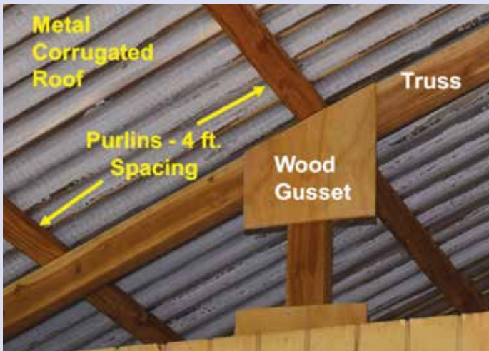
Figure 4-3. On top of the concrete structural bond beam is commonly a wood top plate, consisting of 2 inch by 4 inch lumber. On top of the wood plate are the trusses. To prevent wind damage during a storm, there must be a strong connection from: (a) the wood top plate to the structural bond beam; (b) the trusses to the wood top plate; (c) purlins to the trusses; and (d) metal corrugated roof to the purlins.
