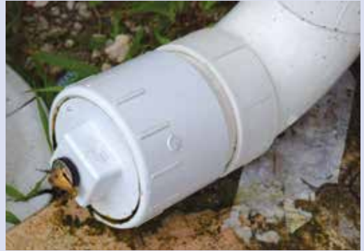
Figure 4-53. At the end of the diversion pipe is a small drain hole that allows the first flush water to slowly drain out so that the diversion pipe is empty for the next rainfall event. In addition, the threaded cap allows for the periodic removal of leaves or other debris.
