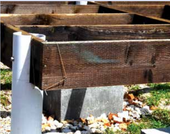
Figure 4-36. Example of ACZA wood suitable for use in the marine environment. Note the cuts or incisions on the surface to increase penetration of the chemical treatment. Because the chemicals in this wood are very corrosive, as well as the marine environment itself, stainless steel fasteners are used to attach the column to the wood joists (support for the flooring). Photo courtesy of Ben Chutarro.
