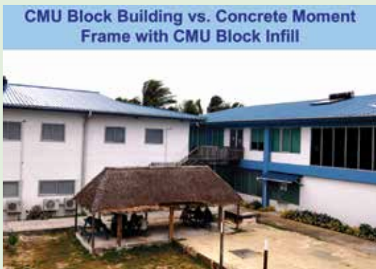
Figure 3-5. The building on the right has a Concrete Moment Frame as shown by the blue columns and beams and CMU block infill (Administration Building at CMI). Compare that with the building on the left with only CMU blocks (Tole Mour Hall at CMI). The building on the right is stronger because of the Concrete Moment Frame.
