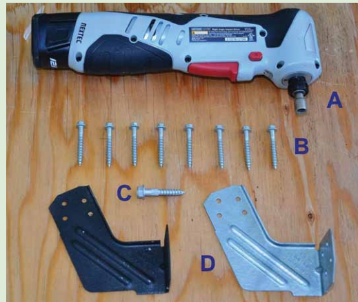
Figure 4-8. For the simple installation in Figure 4-7, a right angle impact driver (A) is used to install the manufacturer's specified connections. Eight Simpson #10 wood screws with 1.5 inch length (B) are used for the top tab (roof connection) and the bottom tab (wall connection). In addition, one ¼ inch Simpson screw with 1.5 inch length (C) provides connection from the trim board to the wall. The HPT clip (D) is shown in its original state, and also primed and painted for the use with black rafters.
