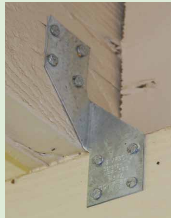
Figure 4-4. This is an example of retrofitting an existing house, originally built without hurricane clips. The popular H3 clip is used here; four nails attach the clip to the roof (truss-rafter) and four more nails attach to the wall or top plate below. For a retrofit, the clips are exposed on the outside of the house, therefore, both the clip and fasteners should be corrosion resistant and painted to blend with the exterior of the house. With the correct clip and nails you could perform the work or, if you prefer, hire a licensed contractor. 23
