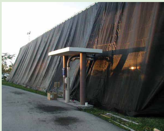
Figure 4-23. Hurricane screen, mesh, or fabric consists of woven polypropylene, which is a plastic polymer. The screen can cover large areas and provide protection to windows with unusual configurations. Light can pass through the fabric so that the area inside is not totally dark. Photo courtesy of the Department of Emergency Management, City and County of Honolulu.
