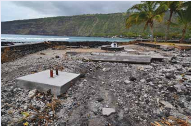
Figure 2-2. The tsunami generated from the March 11, 2011 earthquake off Japan damaged many residences in Kealahou Bay on the island of Hawai'i. The house on this empty lot was swept into the bay.
