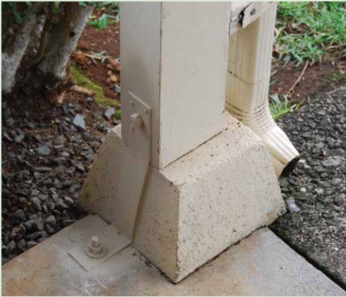
Figure 4-6. In some retrofit examples, it is possible to tie a portion of the house to the foundation. Here, a metal strap connects the vertical post to the foundation, which attempts to finish the continuous load path connection from the roof to the foundation. Photo courtesy of Hurricane Protection Services.
