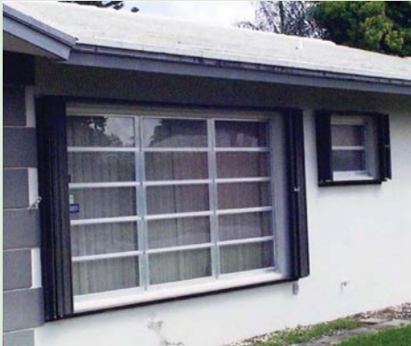
Figure 4-12. For deployment during a storm, the panels unfold accordion-style and extend toward the center of the window along pre-installed tracks. Photo courtesy of the Department of Emergency Management, City and County of Honolulu.
