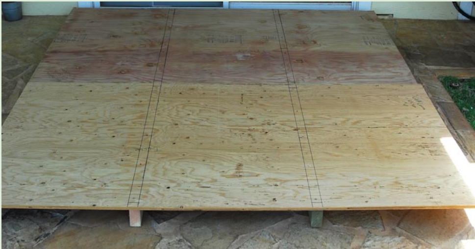
Figure 4-27. During assembly of the shutters in Figure 4-26, the two panels to be joined sit atop the 2 by 4's. The outline of the 2 by 4's and all screw locations are marked on the panel. Panels should be cut, labeled, and marked as to all fastening locations before hurricane season. The panels can be quickly attached with wood screws drilled from the plywood panel into the 2 by 4. The panel is then raised with the end near the window being the pivot point. The panel is then attached to the structural framing of the window as shown in Figure 4-26.
