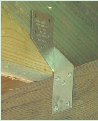
Figure 4-3. This is the popular H2.5 hurricane clip installed during new construction of houses. Five nails are hammered into the lower beam (or top plate) and five more need to be used for the roof (truss-rafter) connection. A hurricane clip is required for each truss-rafter. Upon completion of this structure, the hurricane clip will be hidden from view. This particular clip costs 30 cents. For less than a dollar in material cost, stronger ones can be installed for both new and retrofit applications.
