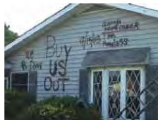
Glenville, DE home after the flood
