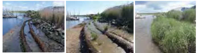
PDE and Rutgers Haskin Lab Living Shoreline Installation. At left: April 2010. Center: June 2010. At right: June 2011.
