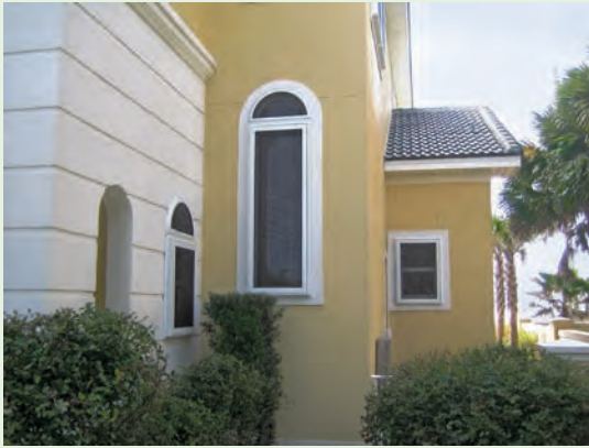
Figure 4-15. In-place stainless steel impact screen protects several windows of a coastal residence. This system requires no deployment and provides shade. Image courtesy of Roll-a-way
