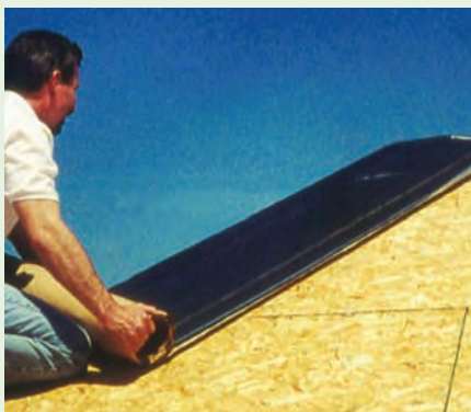
Figure 4-10. Synthetic underlayments are typically made from polypropylene, polyester, or fiberglass fabric, which weighs less than felt building paper, can be manufactured with anti-slip surfaces, and can withstand exposure to the elements for six months. Image courtesy of Carlisle Coatings & Waterproofing
