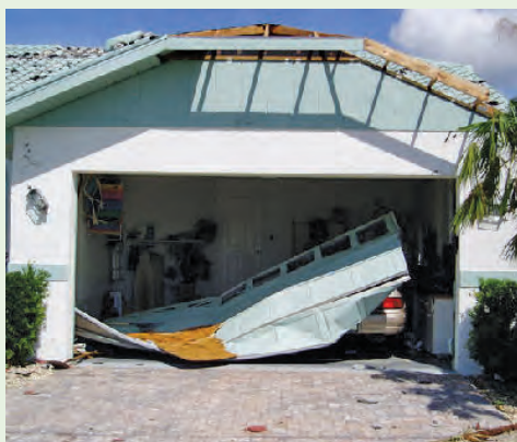
Figure 4-22. Because of their width, double-wide garage doors are more susceptible to wind damage than single doors. The wind can force it out of the roller track, especially if the track is lightweight or some of the anchor bolts are not in place. This occurs because the door fails under excessive wind pressure. You should reinforce your garage door by installing horizontal and/or vertical bracing onto each panel, using wood or light gauge metal girds bolted to the door mullions. You may also need heavier hinges and stronger end and vertical supports for your door. 4.12 Image courtesy of Florida Hurricane Depot
