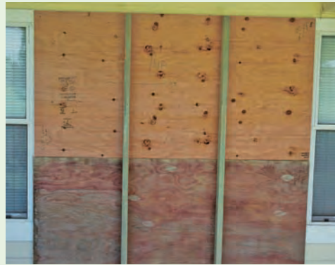
Figures 4-20 and 4-21. Not only is it necessary to install plywood opening covers correctly, it is also important to correctly label them and store them away from heat and humidity. Images courtesy of Dennis Hwang
