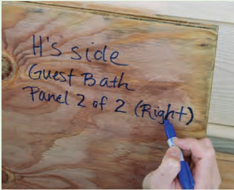
Figures 4-20 and 4-21. Not only is it necessary to install plywood opening covers correctly, it is also important to correctly label them and store them away from heat and humidity. Images courtesy of Dennis Hwang
