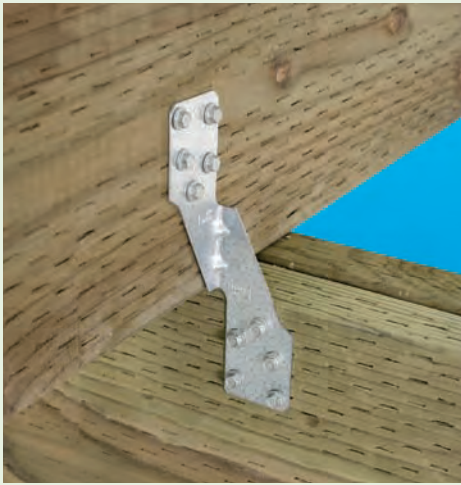
Figure 4-8. This is the popular H2.5A hurricane clip installed during new construction of houses. Five screws are driven into the lower beam (or top plate) and five more are used for the roof (truss-rafter) connection. A hurricane clip is required for each truss-rafter. Upon completion of this structure, the hurricane clip will be hidden from view. This particular clip costs 30 cents. For less than a dollar in material cost, stronger ones can be installed for both new and retrofit applications. Image © 2012 Simpson Strong-Tie Company Inc.
