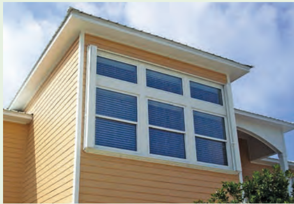
Figure 4-12. Accordion shutter (shown in the open position) installed over a large window of a coastal home. Shutter has been installed to allow deployment from inside the home. Image courtesy of Roll-a-way
