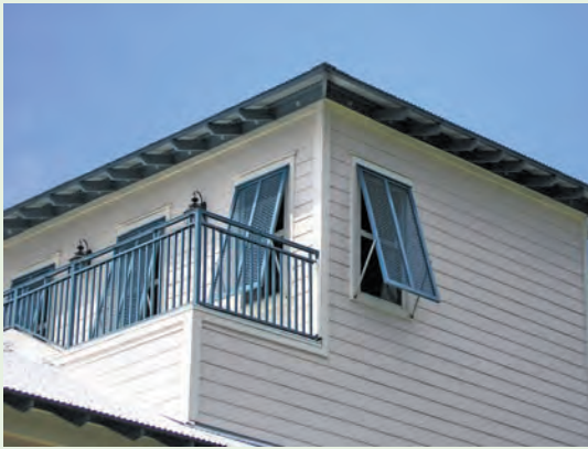
Figure 4-13. Bahama shutters made from durable extruded aluminum components add “islands” flair to a home and provide effective opening protection. Image courtesy of Roll-a-way
