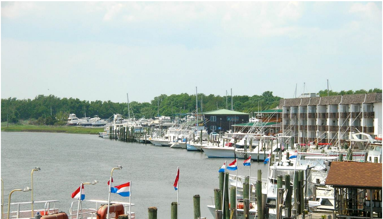
Figure 1.2: Lewes Harbor as viewed from Savannah Road Bridge.
