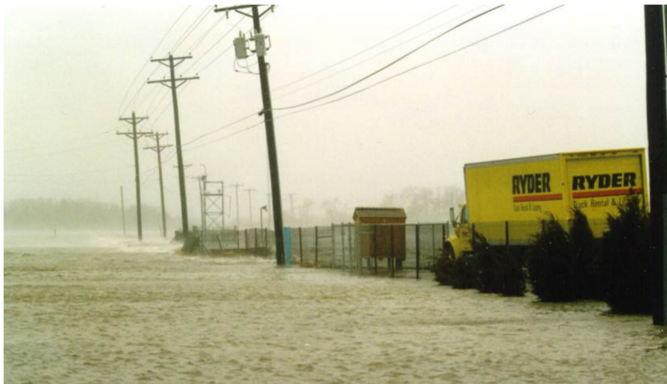
Figure 5.1: Flooding on Pilottown Road during 1998 storm.
