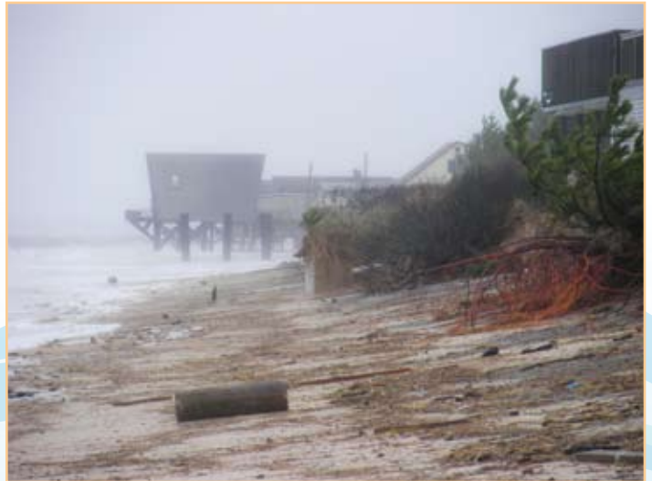
Broken tanks, pipes, and distribution boxes become waterborne debris, which can cause damage to pilings and adjacent structures.
