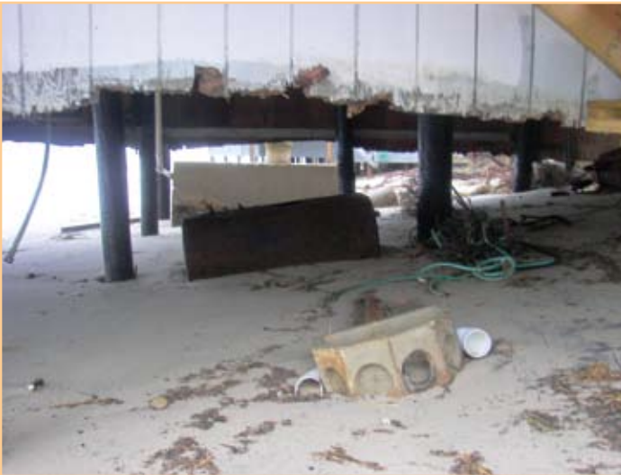
A damaged septic tank can leave a dwelling uninhabitable and vulnerable to future storms.
