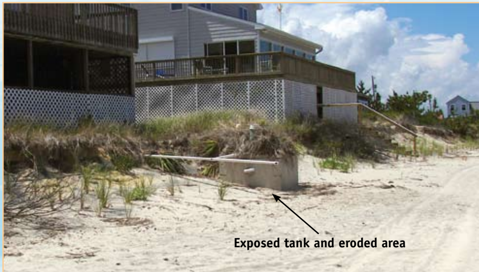
A damaged septic tank can leave a dwelling uninhabitable and vulnerable to future storms.
