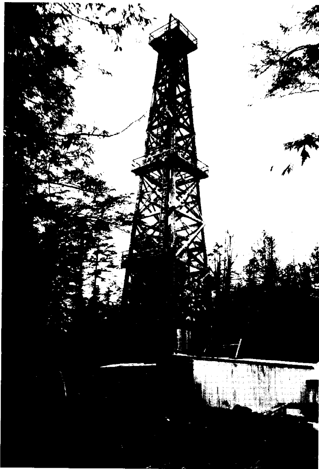
Wooden derrick of the Sims No. 1 well, circa 1931, drilled near the Jefferson oil seep in Jefferson County. Numerous exploratory wells have been drilled in this area and elsewhere on the western Olympic Peninsula and adjacent continental shelf. Photograph courtesy of Jones Photo Company, Aberdeen, Washington.
