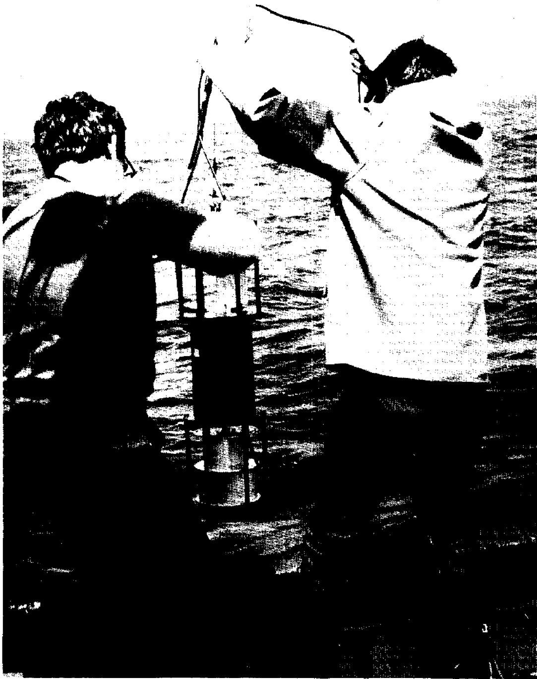
FIGURE #7 Bendix Savonius Rotor Current Meter being lowered into Vineyard Sound by U-M students.
