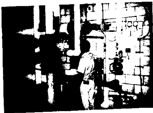
FIGURE 2. "Karbate" heat exchangers in new laboratory. Seawater passes through "Karbate" tubes surrounded by a steel jacket through which hot water from the furnace passes.
