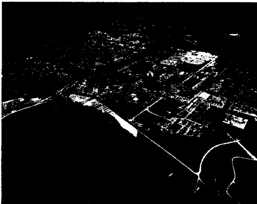
Aerial view of Plant B, Texas Division of the Dow Chemical Company, Freeport, Texas
