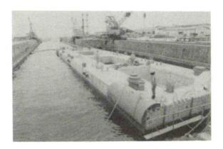
Photograph 5 Floating Breakwater just after joined in the dock
