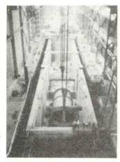
Fig. 3. Large Cavitation Channel Under Construction
