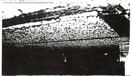
Figure 9 Outward appearance of the Bottom Shell Plating after peeling by robots
