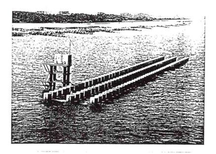
Fig. 5. Slit-type large-scale offshore breakwater (PBS method); the Suruga Coast
