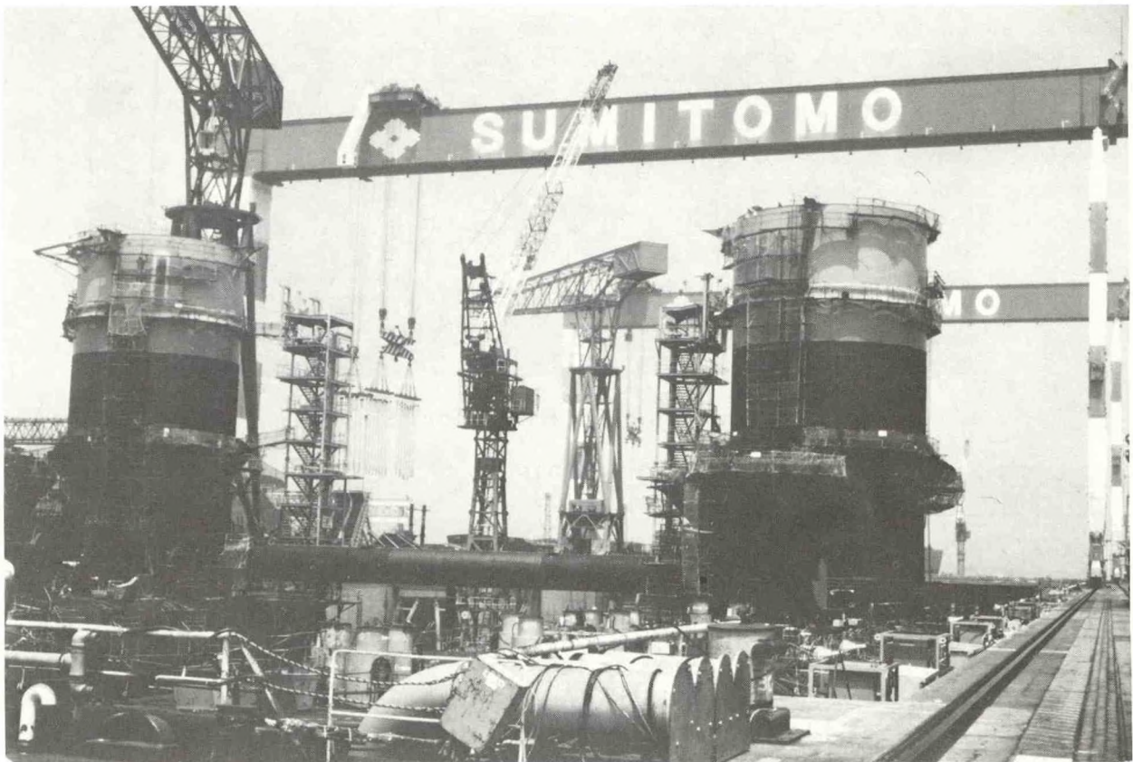
Offshore Drilling Platform Under Construction at Oppama Shipyard of Sumitomo Heavy Industry
