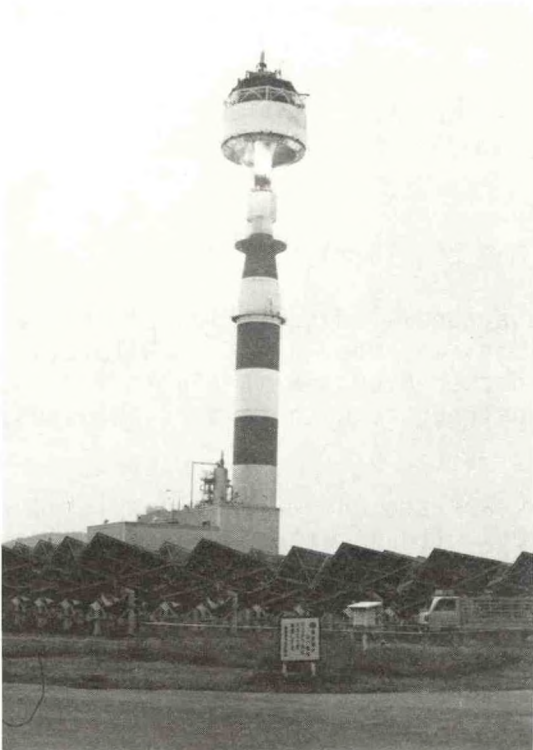
Solar Energy Pilot Plants, Nio-cho, Japan Left: Central Receiver System. Right: Plane Parabolic System.
