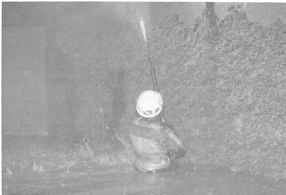
Waist-deep in water, this Detroit Edison worker is using high pressure water to remove zebra mussels from water intake pipes. To prevent this biofouling, Sea Grant provides electric power companies with the best available technology to manage this problem. Photo: Detroit Edison
