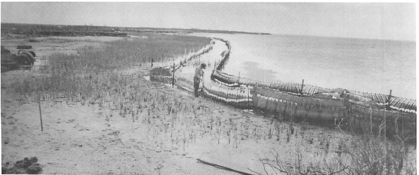
In a shift to "soft" strategies to control beach erosion, a project by Sea Grant uses parashutes to absorb wave action and allow smooth cordgrass to take hold. Photo: Texas Sea Grant
