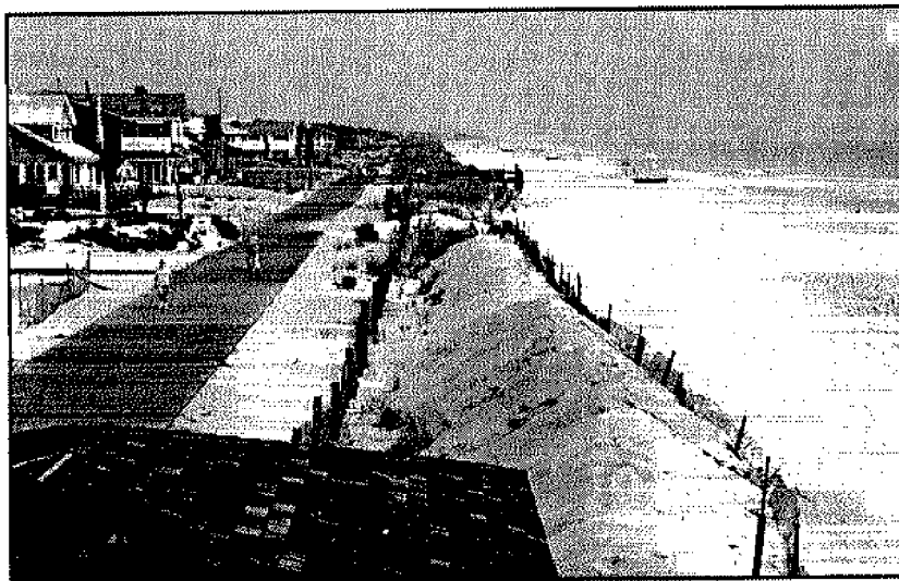
Figure 13. Constructed dune with parallel fencing to define the dune's boundaries. Lavallette NJ
