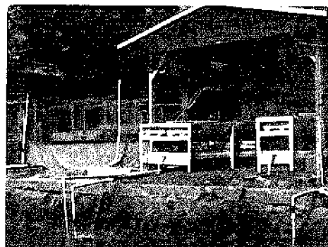
Figure 3. Covered holding facility at Belau Aquaculture in Palau. (Eileen Ellis)
