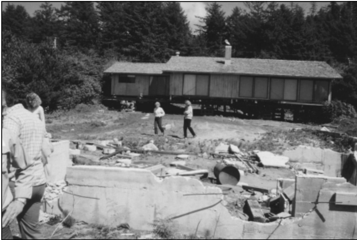
Relocation of existing buildings threatened by erosion is a viable mitigation strategy in many cases, but is rarely used. This house at Cove Beach in southern Clatsop County is an exception (J. Good photo).
