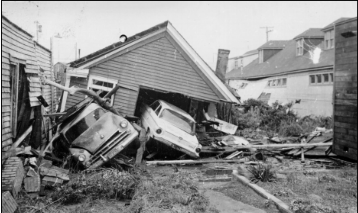
The tsunamis that hit Crescent City, California, following the March 28, 1964 Alaskan earthquake claimed 11 lives and caused more than $7 million in damage (G. Griffin, Crescent City photo).
