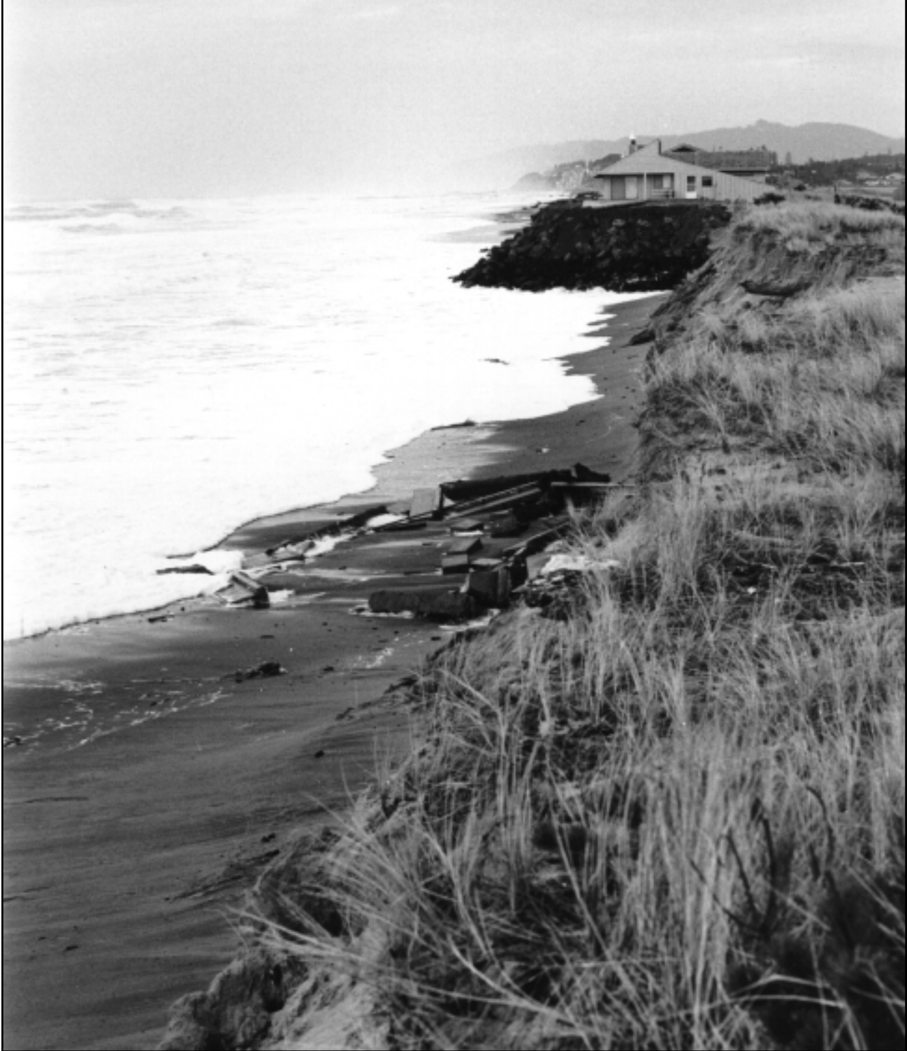
Some erosion events clearly create shore protection emergencies, such as this one on Siletz spit (P. Komar photo).
