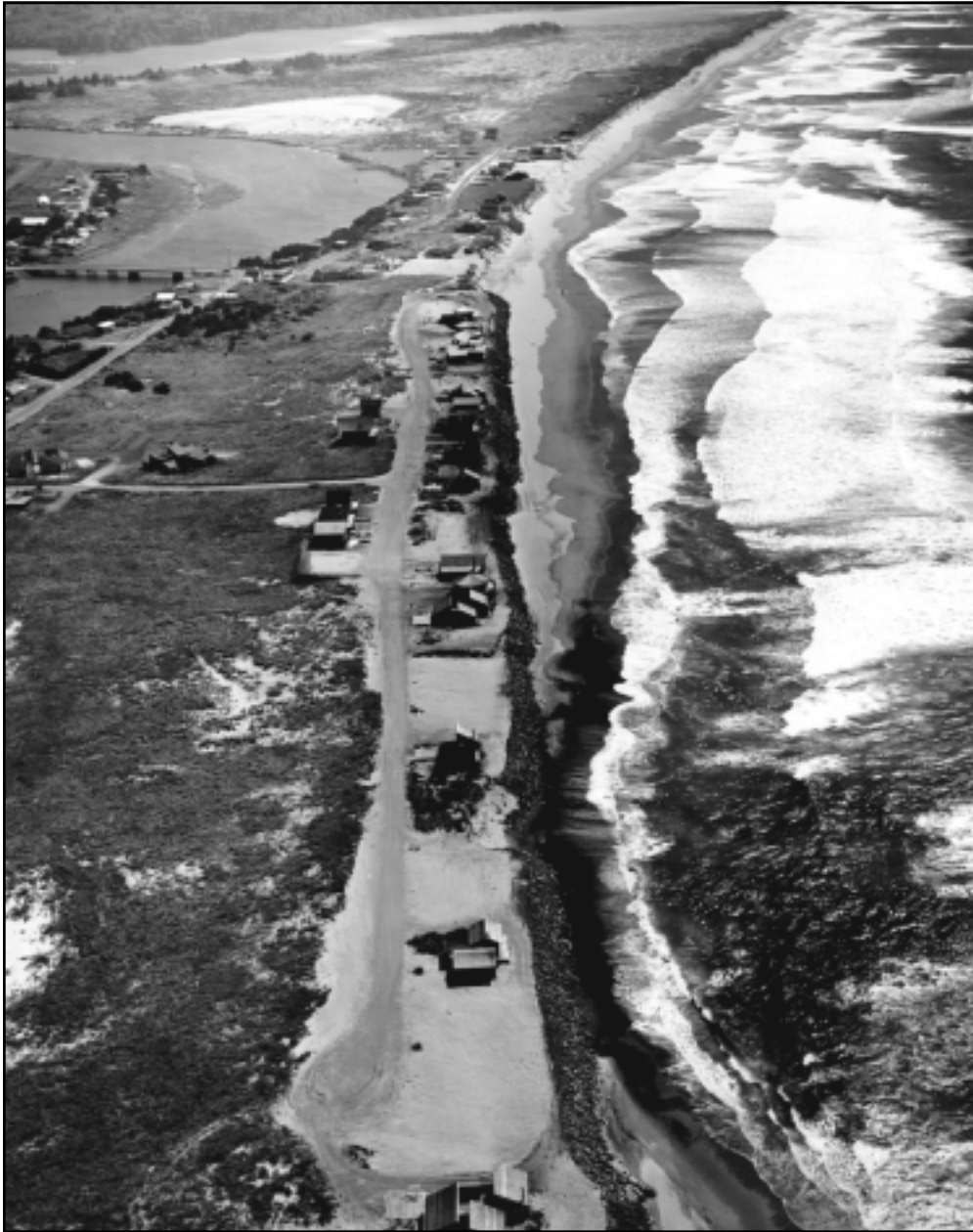
Development continues to fill in on previously subdivided property in Pacific City without regard to obvious erosion hazards; unless the unbuilt lots are abandoned, the only available hazard mitigation is shoreline armoring with riprap (ODOT photo).
