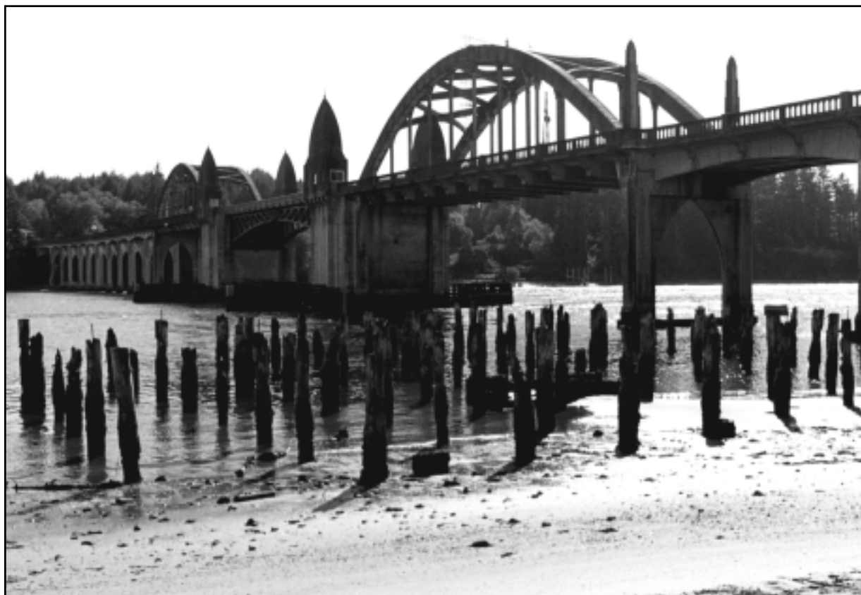
Many older bridges along the coast, such as this one at Florence, would likely be severely damaged by a large CSZ earthquake (J. Good photo).
