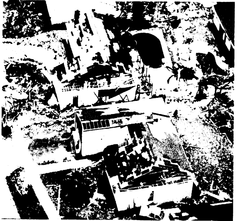
Figure 22. Family home damage from Andrew (U.S. Army Corps of Engineers, 1993).
