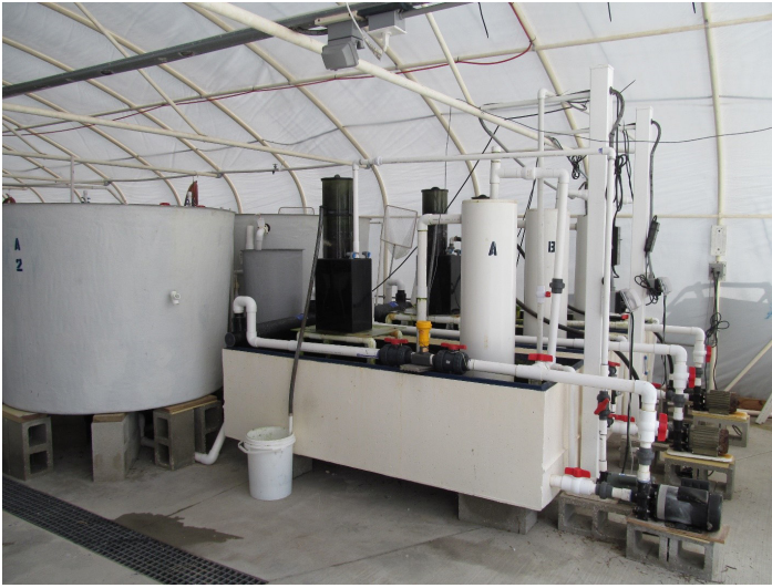
Figure 10. Recirculating system used in the culture of marine ornamental fish. Credits: UF/IFAS Extension
