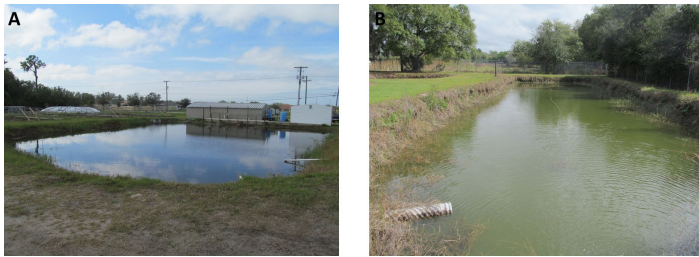
Figure 9. Detention pond (A) and retention pond (B) at a certified aquaculture facility in Hillsborough County. The detention pond discharges through a control structure to a county ditch in the background. The retention pond has no off-site effluent discharge; however, an inflow pipe from an interior ditch is seen in the foreground. The retention pond is underlain by permeable soils and receives little effluent (effluent pipe seen in foreground) from pumped ponds, making this solution feasible.
