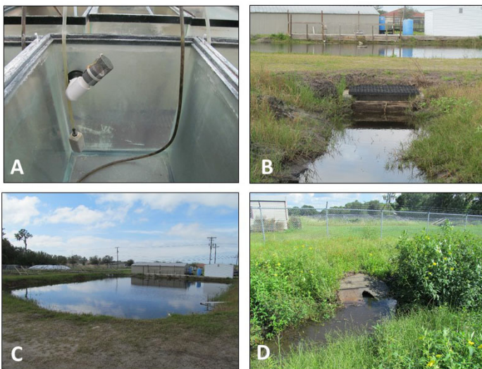
Figure 3. Critical Control Points (CCPs) to prevent non-native species escape at an example facility. A. Screen systems to retain fish inside of greenhouse. B. Control structure separating interior ditch from detention pond. C. Detention pond stocked with predatory fish. Has a control structure as outlet to county ditch. D. Discharge to county ditch.
