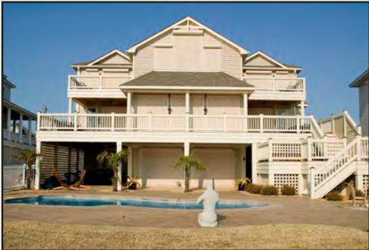
Figure 4-2: Coastal home protected with roll-down shutters on all windows and doors. The shutter is held in place by vertical guide tracks and can be deployed manually or with integrated electric motor. (Source: Roll-a-way/QMI)
