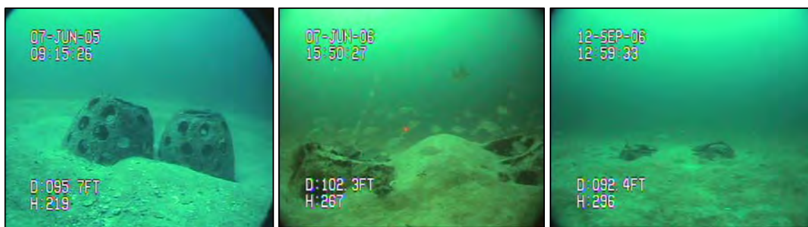
Figure 5.2. Example of subsidence of artificial reef material into soft sediments (Photographs courtesy of FWC).
