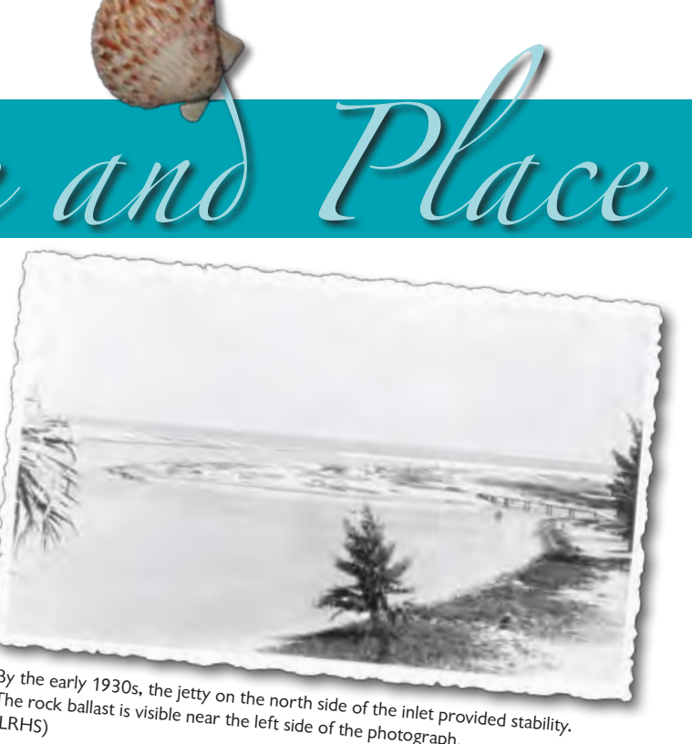
By the early 1930s, the jetty on the north side of the inlet provided stability. The rock ballast is visible near the left side of the photograph. (LRHS)
