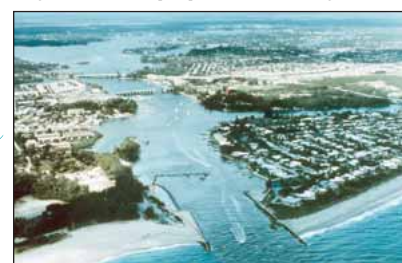
In the foreground of this 1997 aerial photograph, a dredge pump discharges material from the "land trap" in Jupiter Inlet and deposits it on the beach south of the inlet. To the west, beyond the bridges, are the Loxahatchee River Central Embayment and the river's North and Northwest Forks. Photo credit: National Oceanographic & Atmospheric Administration Photo Library (Mrs. Marge Beaver, photographer)
