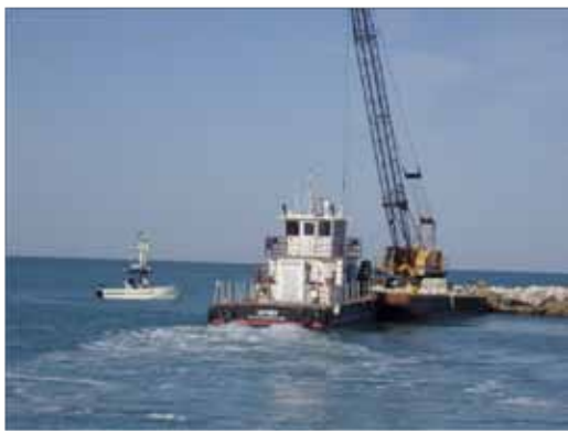
Marine Patrol ensuring safety during Venice Inlet jetty repair operation.
