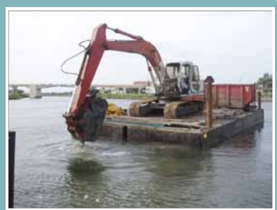
City of Venice boat ramp restoration.
