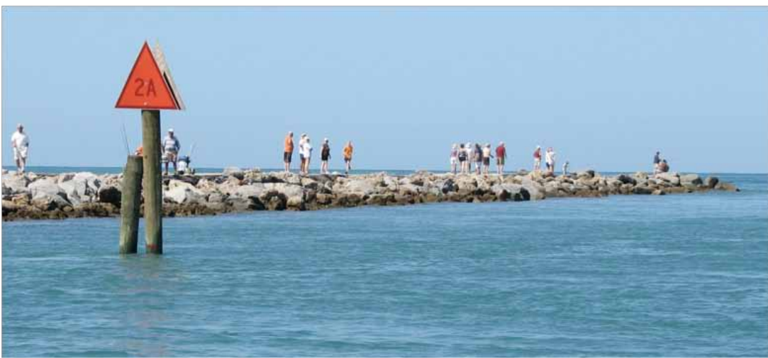
Venice Inlet jetty following repair.
