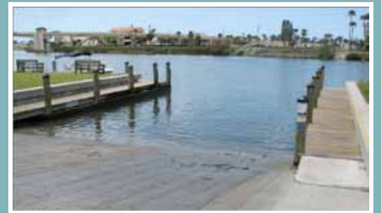
City of Venice boat ramp after restoration.
