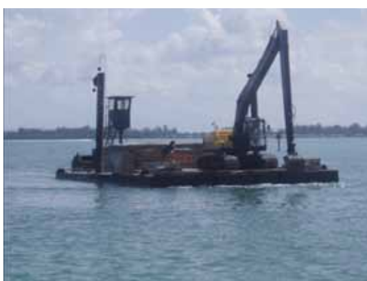
WCIND-managed dredge operation on the GICW.
