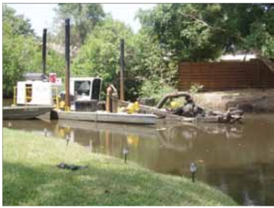
Dredge operation, managed by WCIND, maintaining a secondary channel waterway.
