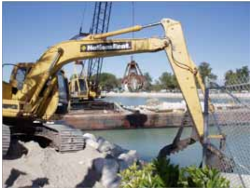
Venice Inlet jetty being repaired after Hurricane Ivan.
