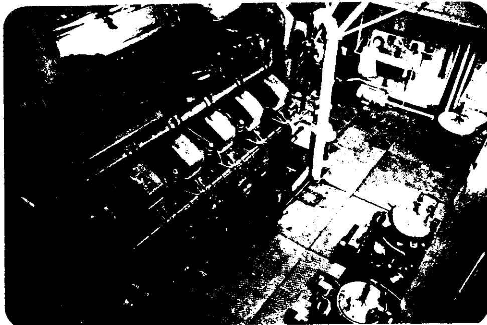
S.E.M.T. Pielstick 12 PA6 V280 heavy fuel engines aboard Great America
