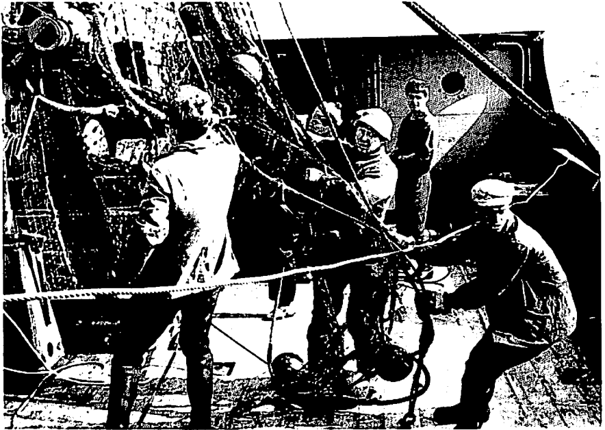
Fig. 7. Crewmen aboard a Soviet trawler prepare to rig a "herring trawl" for fishing. The design of this net has made it a very efficient piece of gear.
