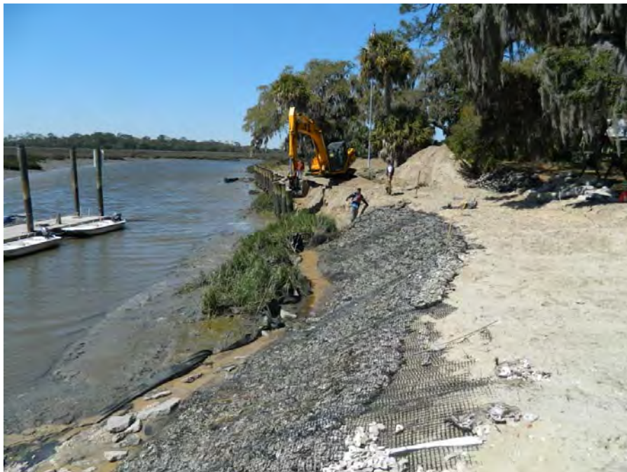
Figure 16. West side of living shoreline March 2013, Little St. Simons Island, GA
