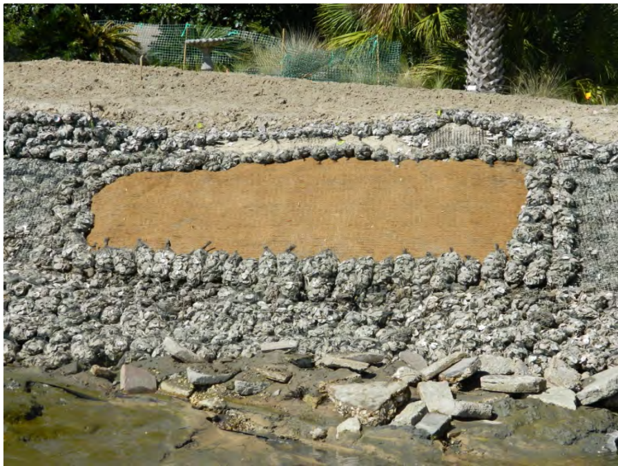
Figure 9. Patch for marsh grasses to be planted into the living shoreline, Little St. Simons Island, GA.
