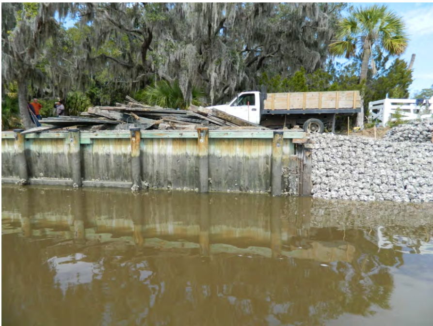
Figure 24. East side of living shoreline March 2013, Little St. Simons Island, GA
