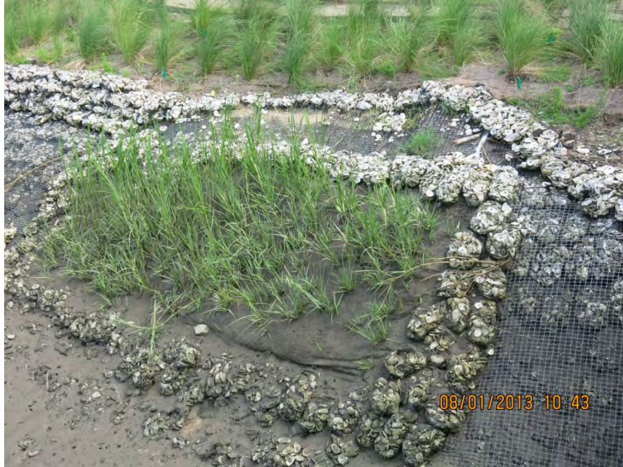
Figure 10. Marsh grasses planted as part of the living shoreline, Little St. Simons Island, GA.
