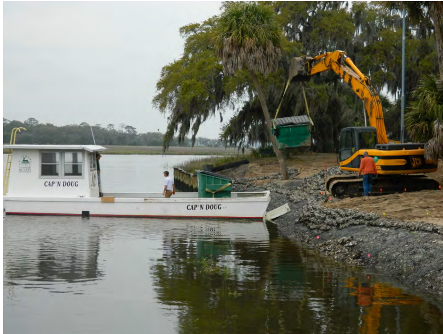
Figure 5. Bagged oyster shell being offloaded to living shoreline site, Little St. Simons Island, GA.
