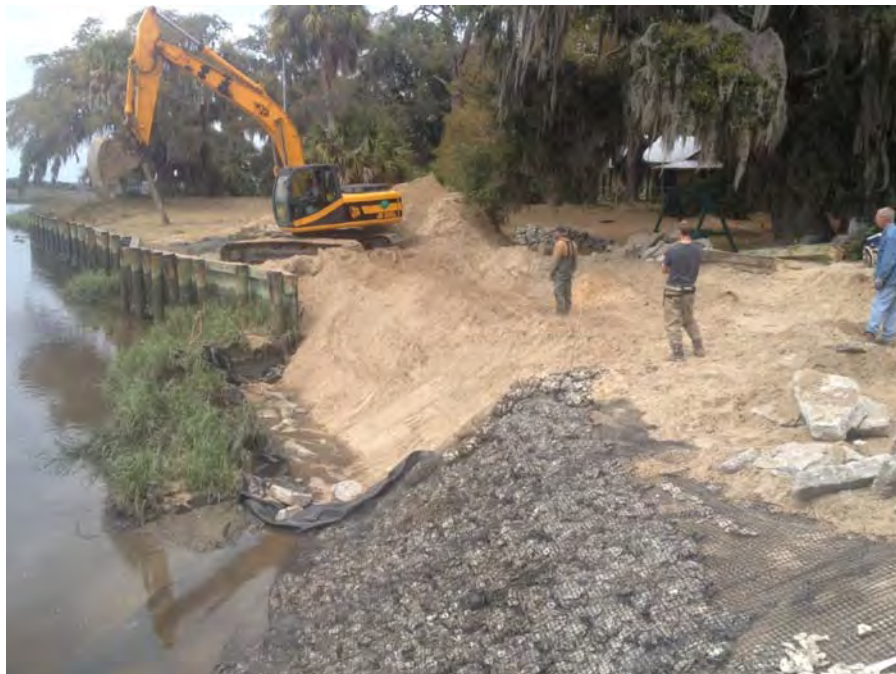
Figure 6. Construction of living shoreline in sections, Little St. Simons Island, GA.
