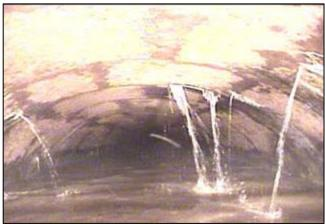
Infiltration into a sewer line. © RedZone Robotics.
