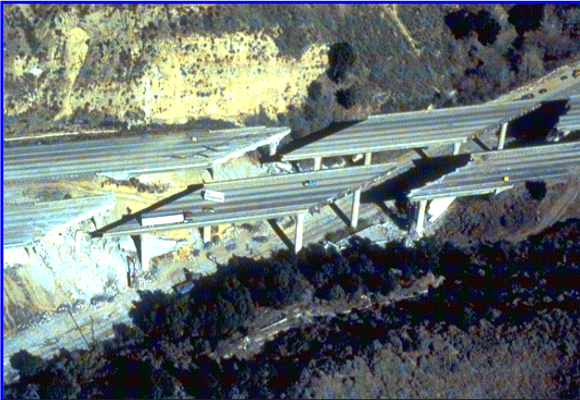
Aerial photo showing damage to a freeway interchange near Los Angeles. The damage was caused by the 1994 Northridge earthquake, of magnitude 6.7. USGS Photo.
