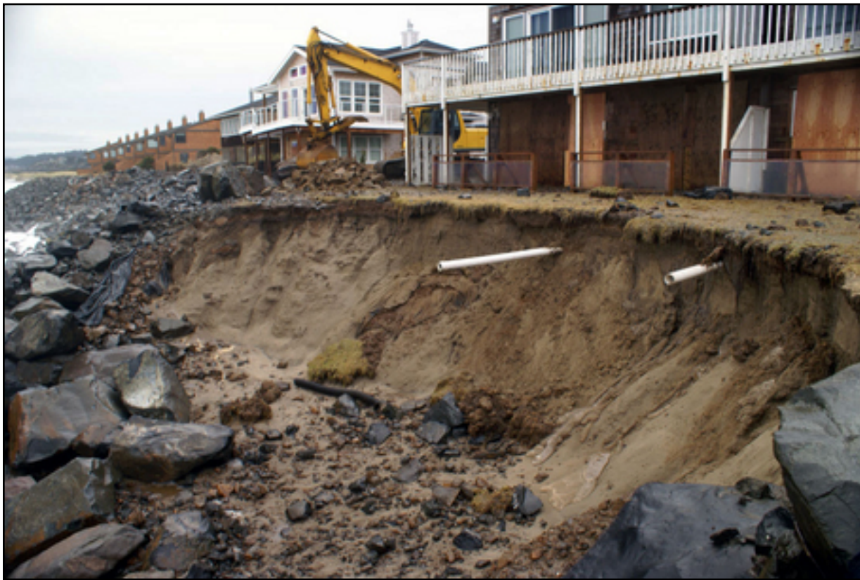
Figure 4. “High surf and the impact on the riprapped Neskowin shoreline on January 9, 2008.” This photo by Armand Thibault appeared in the Oregonian article “State monitoring shifting sands on coast,” March 1, 2009. The exposed area in the foreground was riprapped, but the revetment was damaged by storm waves and was undergoing repairs at the time the photo was taken.
