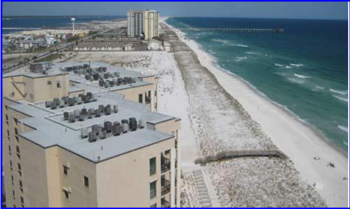
Storm berm constructed at Navarre, Florida, in 2006 to protect the beach and shoreline properties Paden E. Woodruff III, "Providing Protection for the Panhandle," in Coastal Voice: The Newsletter of the American Shore & Beach Preservation Association , September 2010, p. 16.
