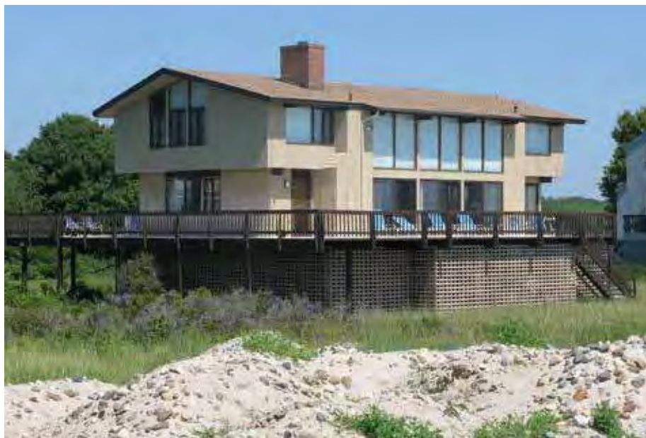
This coastal Maine home was set back behind a berm and raised up on its foundation to offer protection from storm surges and rising seas. (PHOTO: JOE CONE)
