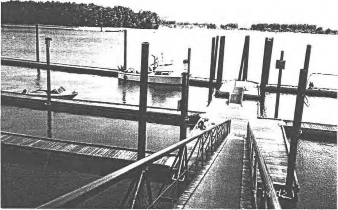
TYPICAL TRANSIENT FLOAT
