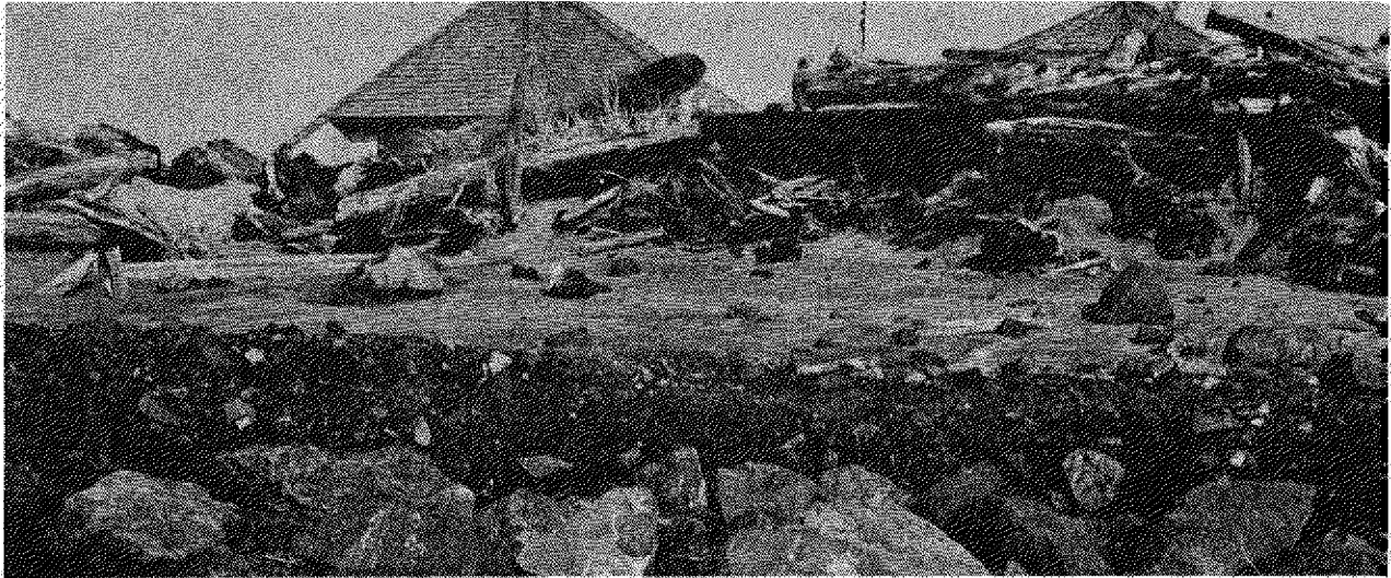
Fig. 8. Erosion of the riprap seaward of the northern most house, photographed on March 20, 1976. It is seen that some of the finer-grained material backing the larger rocks has been eroded away. Waves washed over the riprap, pushing back the drift logs into a pile.
