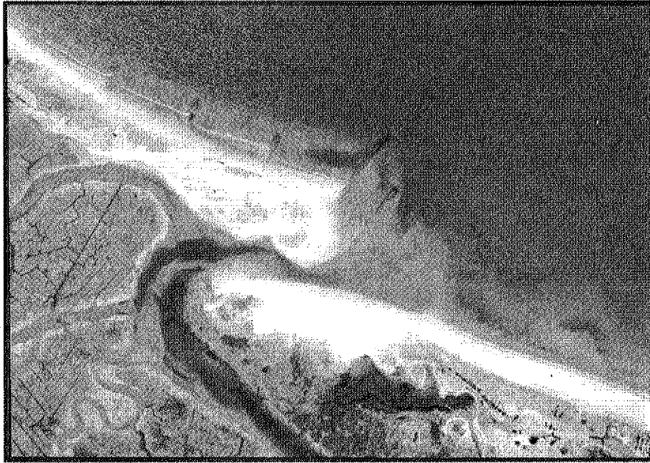
Figure 1. Aerial photograph of Sandwich Harbor Inlet indicating breach from existing structures and thalweg migration to the southeast (2001).
