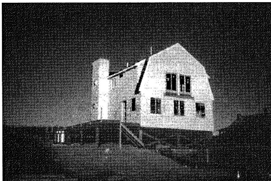
Figure 14. House elevated on open pile foundation
