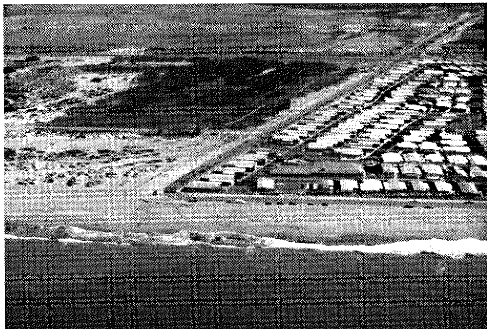
Figure 1. Oxnard Shores, CA, showing elimination of dune to construct a road
