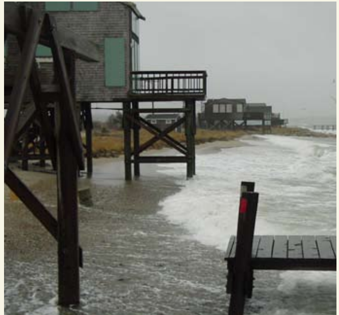
Elevating waterfront structures on open pilings, while protecting the structures from storm waves, will not prevent erosion-related damages.
