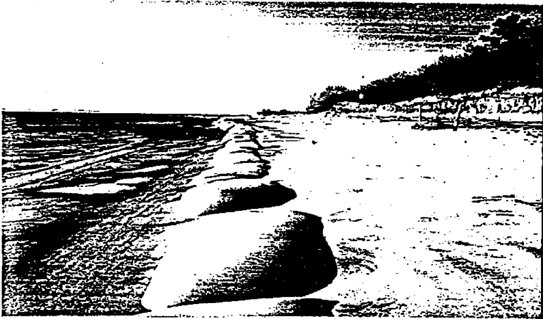
Perched beach project at Morris Island, MA. This photograph was taken after the January storm (1/12/78) which was the only time a perch developed at this site.
