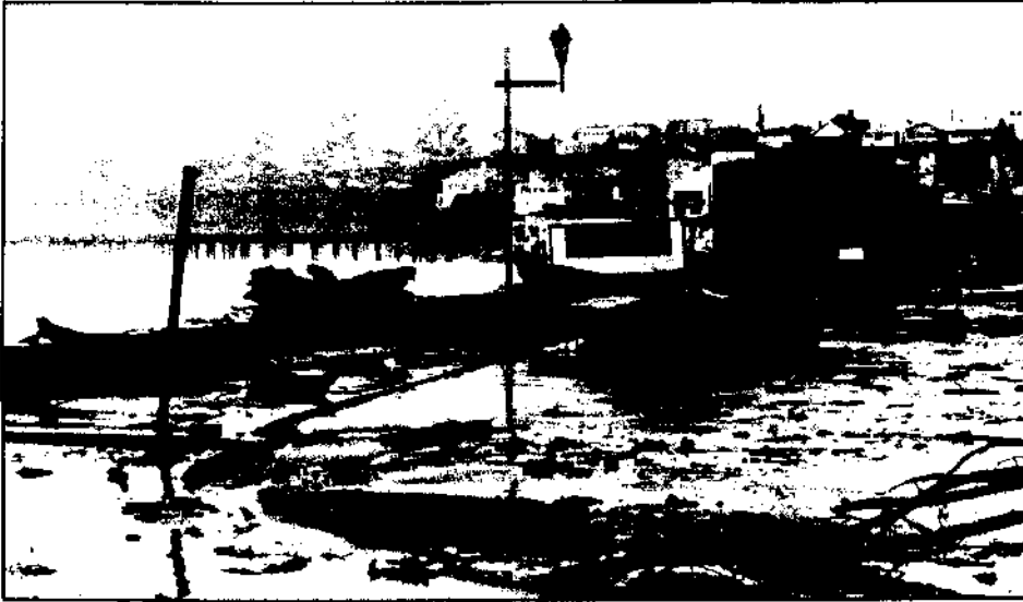
Figure 45 Storm waves overtopped a low concrete seawall in Capitola during the winter of 1983 and washed debris into the streets (Site 19).
