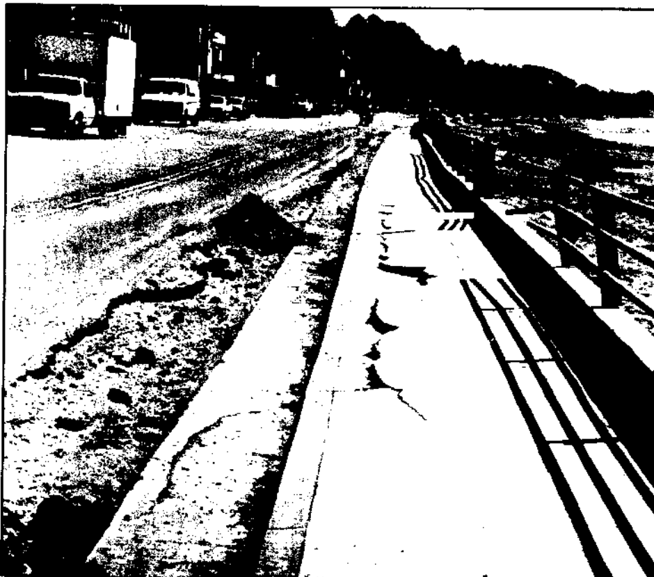
Figure 31 Overtopping of this seawall and clogging of drain system led to piping through underlying fill and collapse of pavement (Site 25).
