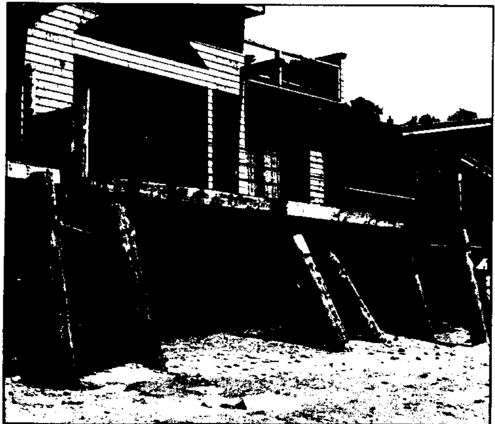
Figure 33 Removal of lagging and collapse of wooden seawall due to scour and wave impact (Site 26).
