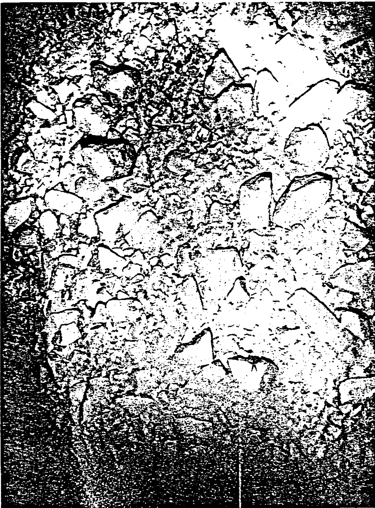
FIGURE 5.41: ROCK DUMPED BY SPLIT BARGE CLOSE UP VIEW SHOWING MIXING OF FINE AND COARSE AGGREGATES
