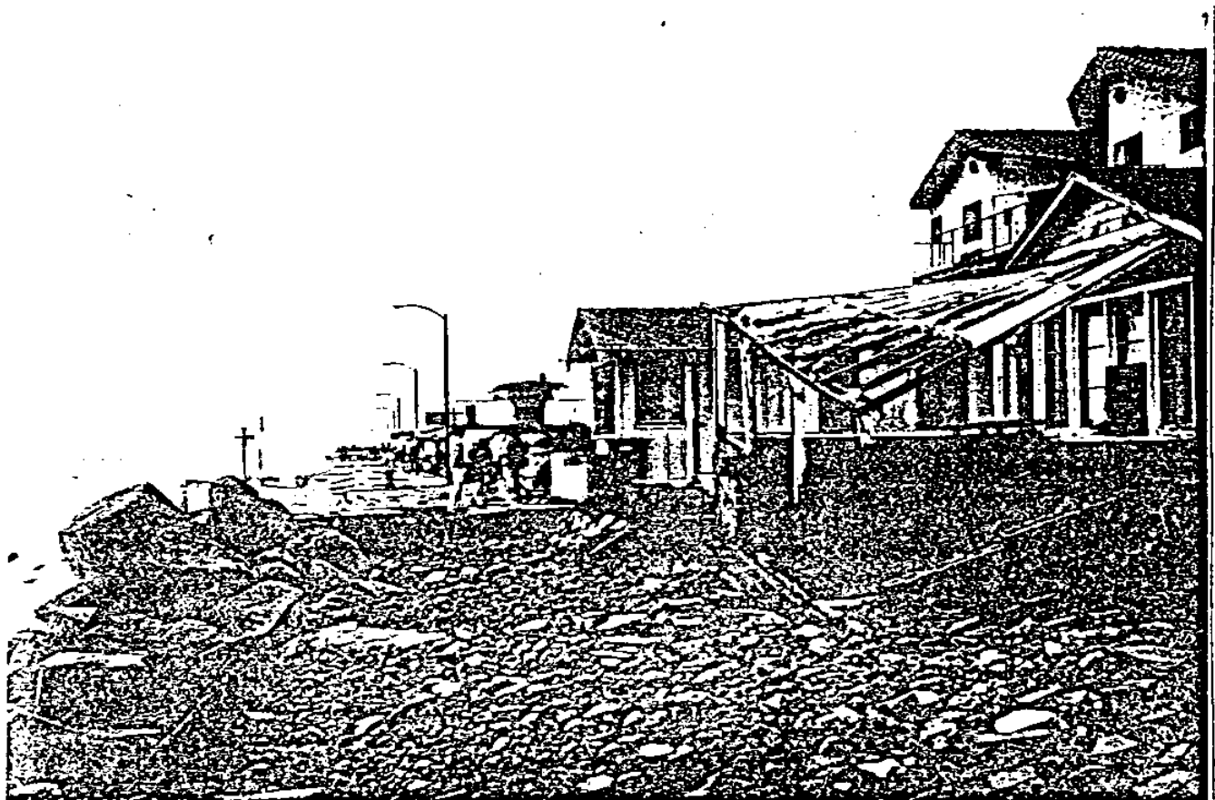
B. (After) Same view in 1980 showing wave and beach cobble abrasion which damaged houses along the shore during storms in Feb. 1980. Property damaged occurred during relatively small (4-6 ft) swell. Photo: Sea Grant, Feb. 17, 1980.
