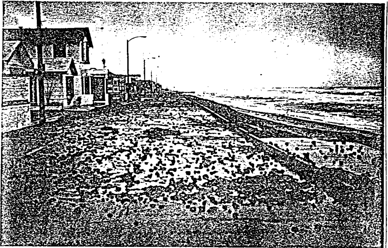
B. March 1978. Same view as Fig. 9.A. Beach cobbles were withdrawn by waves and thrown through the air. Buildings along the shore at Oceanside, Calif. were damaged. Photo: Sea Grant/G. Kuhn, March 4, 1978.
