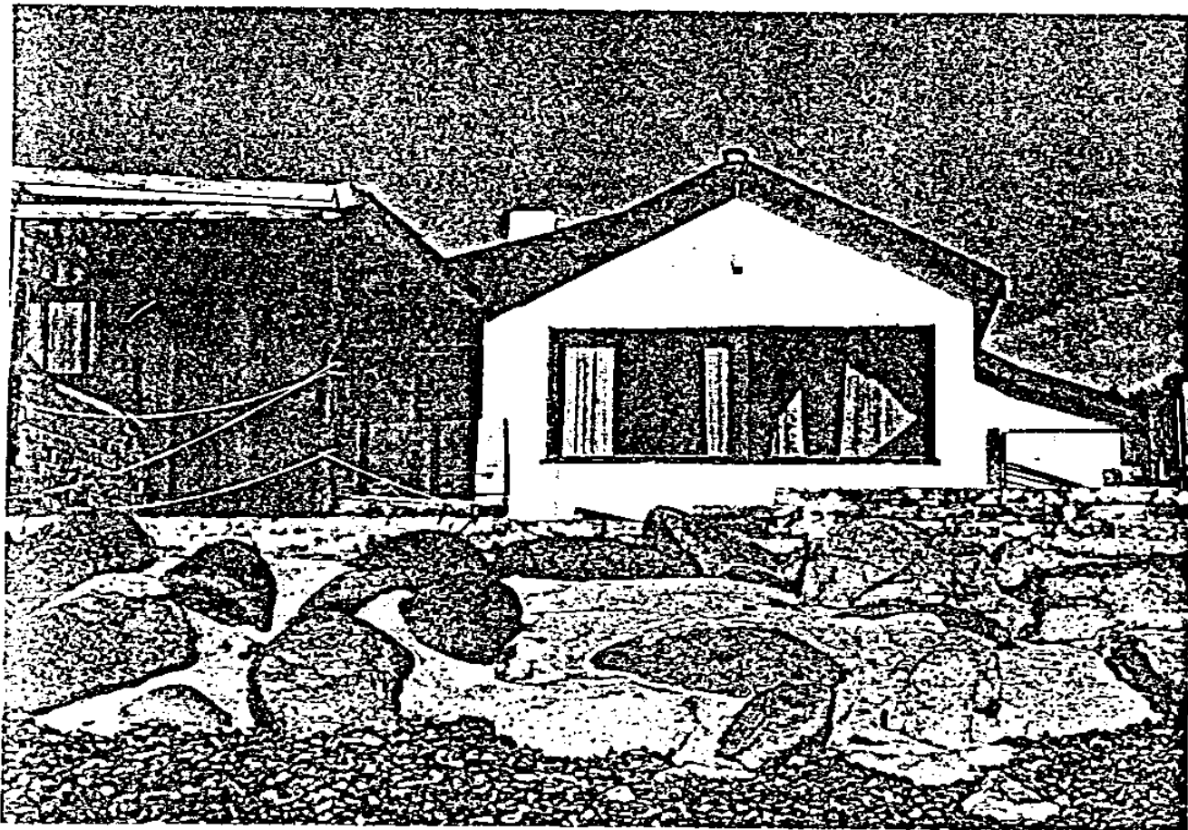
B. 1980. View of house damaged by beach cobbles. Note that windows were broken and roof collapsed as cobbles were withdrawn during storm period of only 1-2-meter waves. Photo: G. Kuhn, Feb. 17, 1980.
