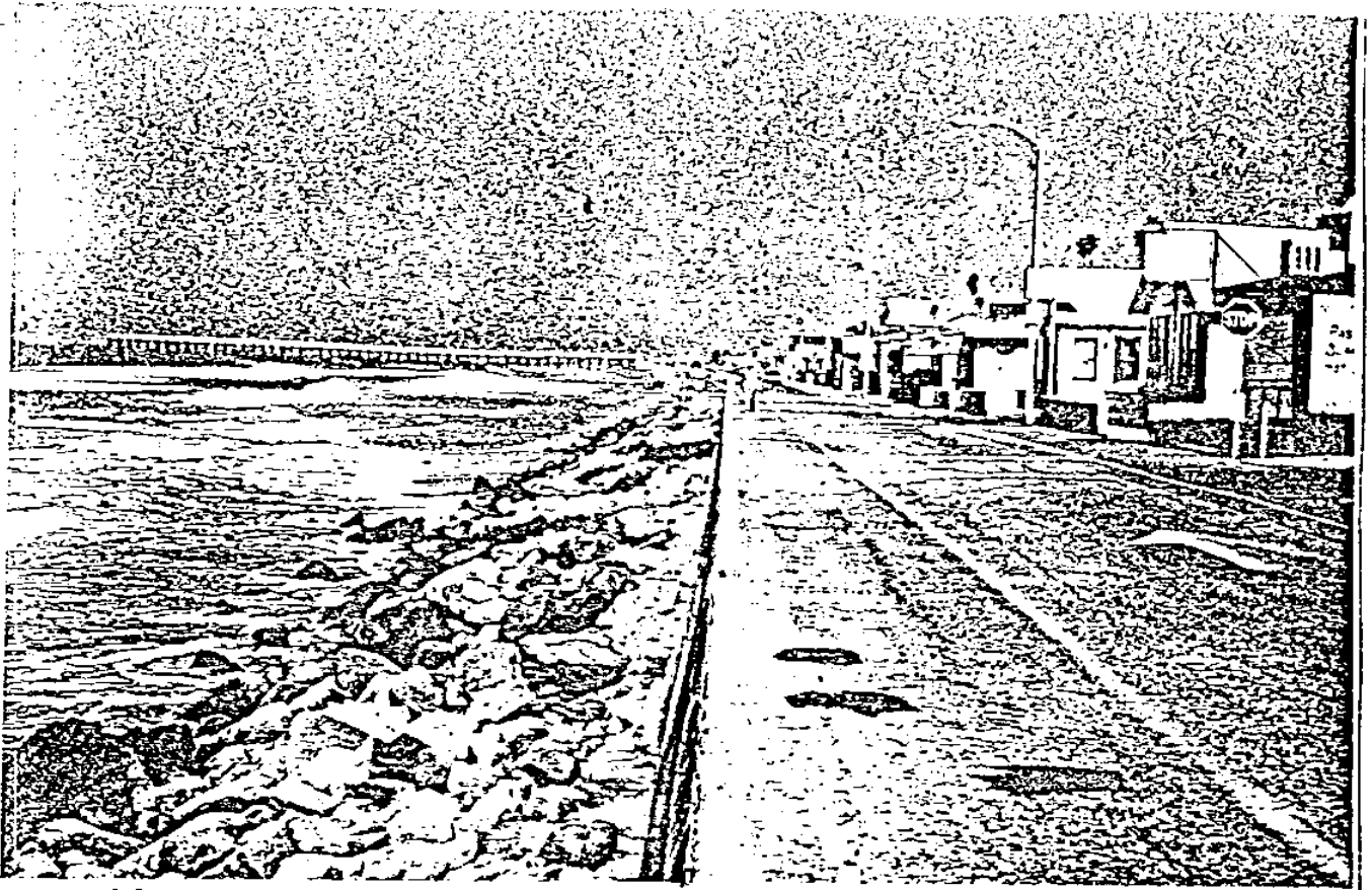
Figure 10. A. (Before) September 1979. View looking north along "The Strand" at Oceanside, Calif. Building and road were constructed on former beach. Riprap fronts and protects concrete seawall and road. Photo: Sea Grant/G. Kuhn, Sept. 22, 1979.
