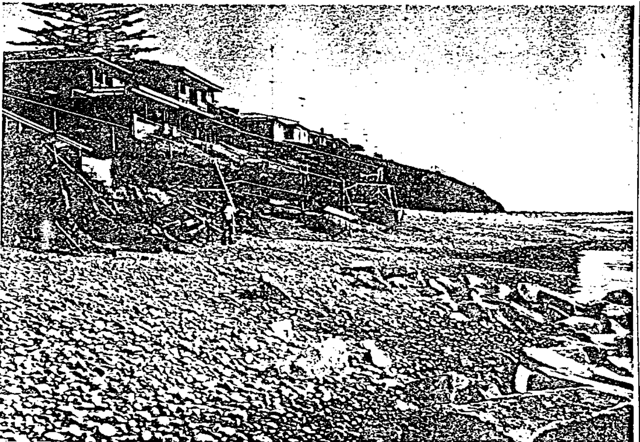
B. March 1978 view of same site as 13.A. Sand levels dipped to very low point and beach cobbles abraded under and around fences, stairways and walls. Photo: Sea Grant/G. Kuhn, March 16, 1978.
