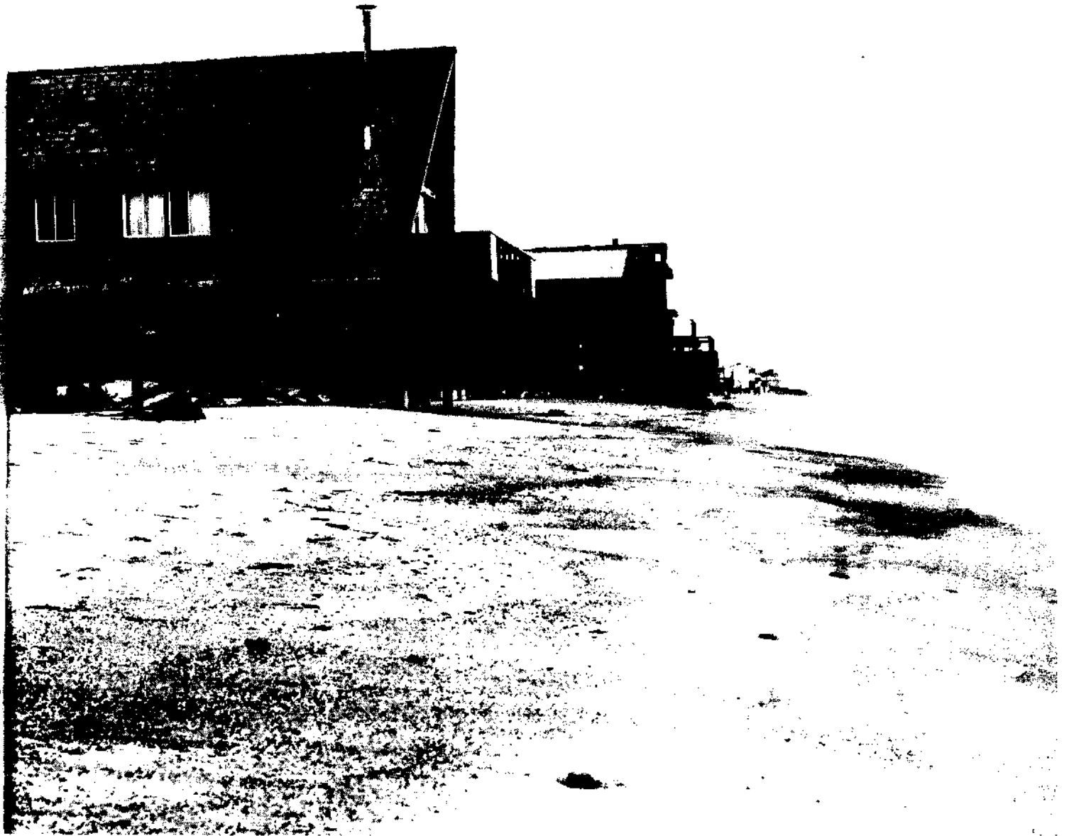
Figure 7.5. Houses at Oxnard Shores, California located on a progressively eroding beach. Note that house in foreground has been raised on girder substructure to avoid wave damage.
